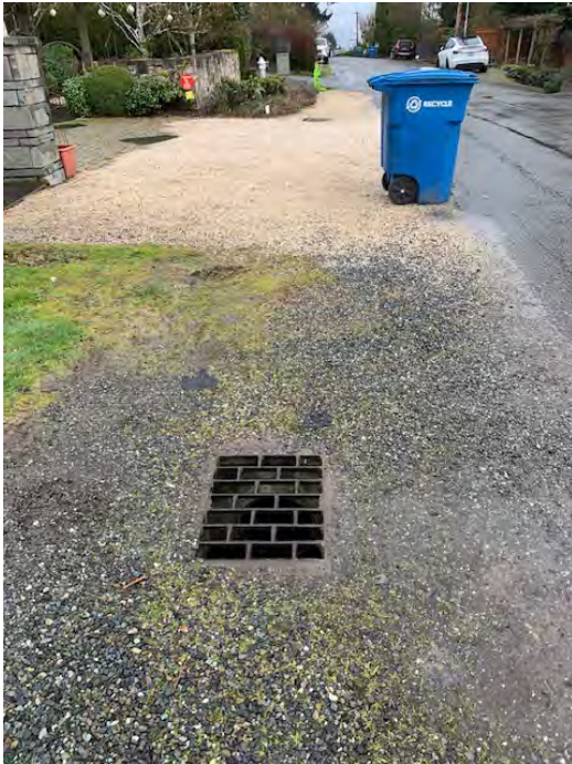
Catch Basin – At point B, Looking Downstream
