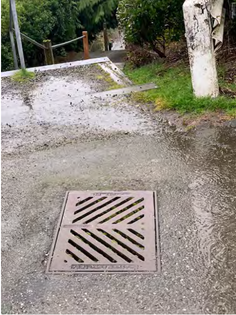
Catch Basin – Point E Top of Trail
