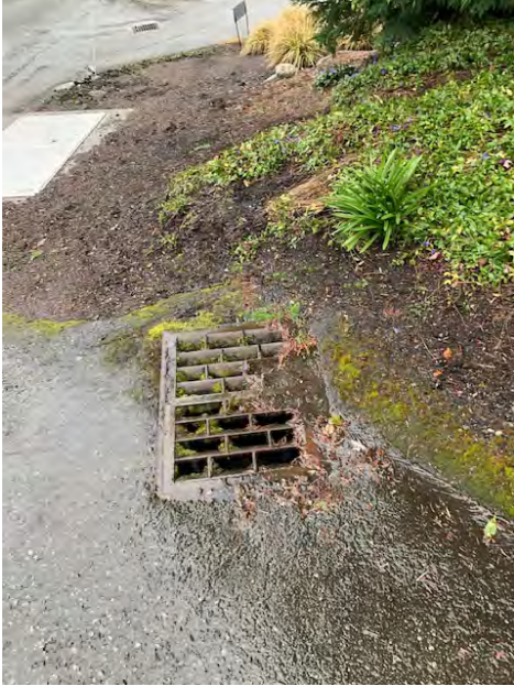
Catch Basin Point H - West of 69 th Ave SE at intersection - Looking West
