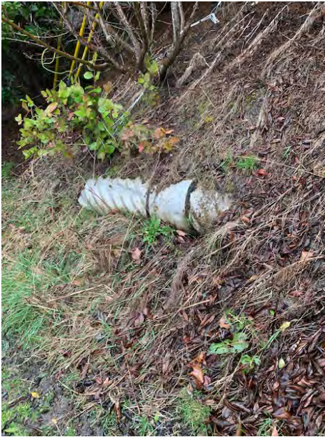
Exposed pipe next to trail near top of trail Point E, no joint leaking
